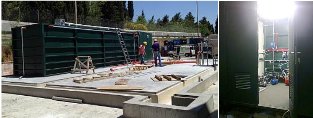
Pictures of indicative compact plants for the treatment of municipal wastewater in hotels and industrial installations.
